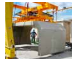
Demoulding, tilting for wall and road segments
