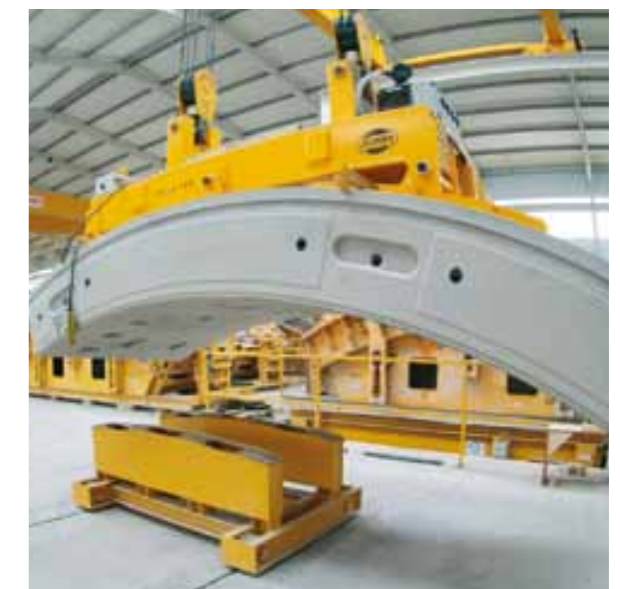
Off line / Vacuum lifter for concrete segment
